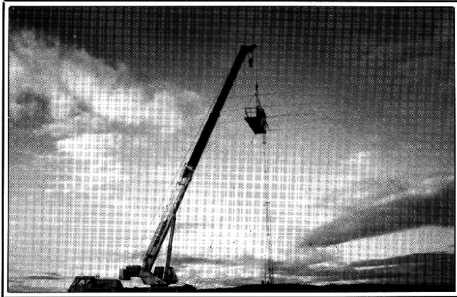
Up goes the 20 meter beam at TF3CW.
