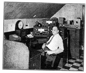
W9EWC made 29,391 points. Butch runs 900 watts input to a pair of 4-125A's modulated by a couple of 304TL's. The exciter is a 310B1, and he also has a 32V2 available. The receiver is a 75A1. For antennas Butch has a 5-element rotary for 10, and a 4-element wide spaced for 20, plus four reversible rhombics.
