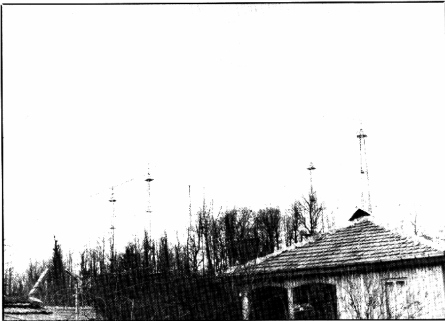
The boys at LZ9A, also LZ2KTS, sported this fine set of antennas—6 elements each on 10, 15, and 20, and 4 elements on 40.
