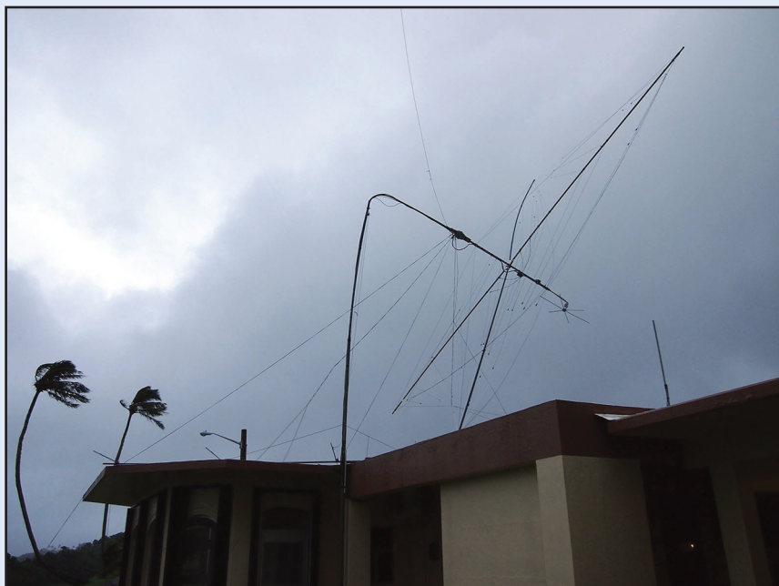
Antenna damage after the tropical storm.
