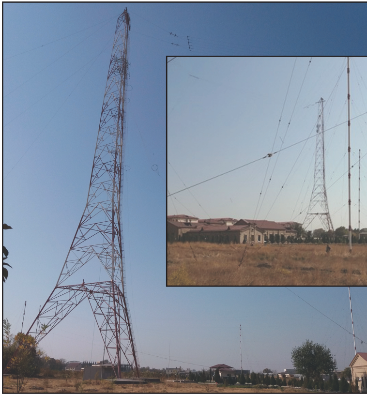
Amazing 7-element wire array on 160 meters at UK9AA.
